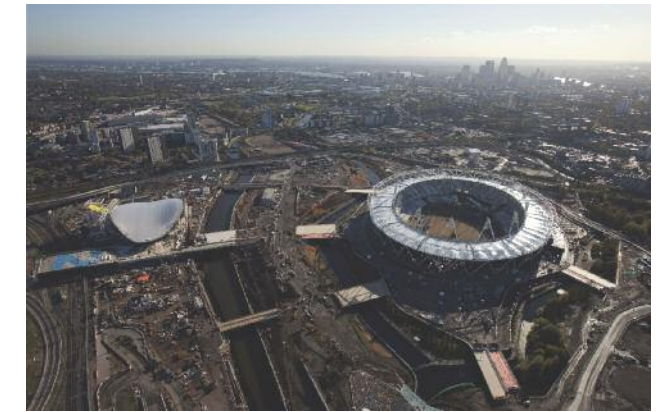
Olympic Stadium. South East facing aerial view of the Olympic Stadium with the Aquatics Centre to the left. Taken on 11 Nov 10 by Anthony Charlton.
