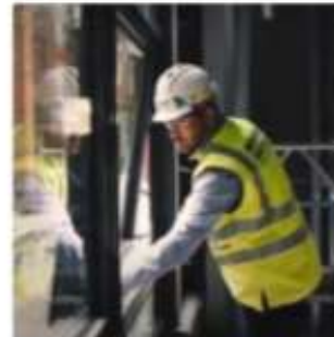
Construction Site Management
