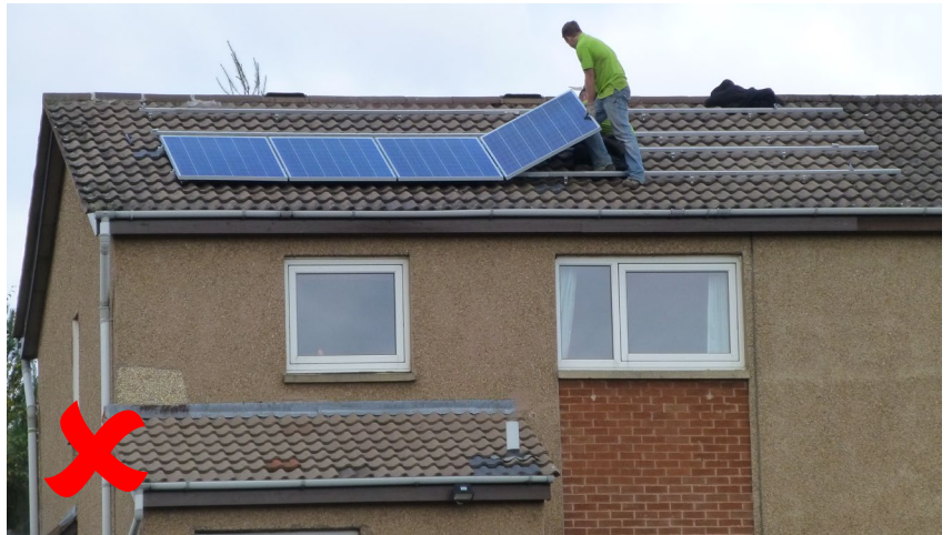
An example of completely unacceptable installation work practices that could easily result in death or serious injury. Unsafe work at height like this would normally lead to immediate enforcement action by HSE inspectors
