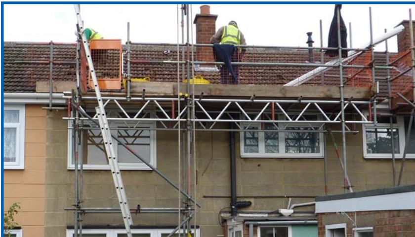
An example showing acceptable edge protection. HSE inspectors would expect to see this standard of protection during solar panel installation.
